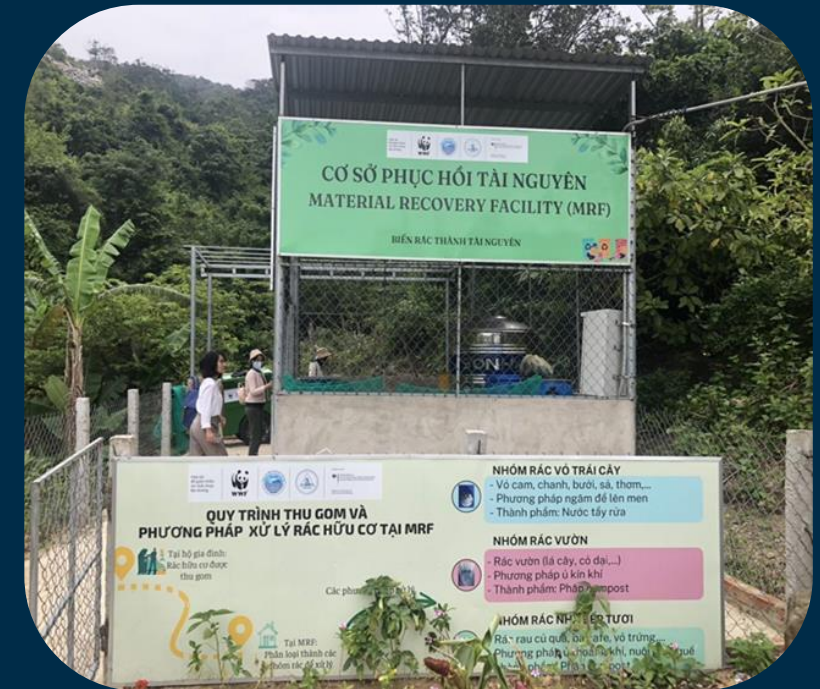
WWF establishment of a small Material Recovery Facility (MRF) in Cu Lao Cham Island, Vietnam
